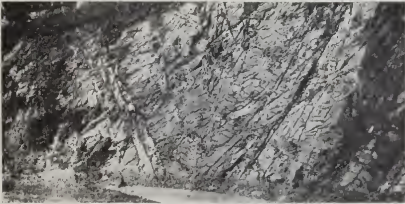
FIG. 1.—Syncline in closely folded strata shown on aqueduct cutting west of Yankee Jim Creek, Upper Yarra District.
